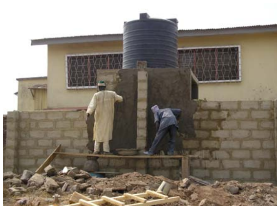
The bricklayers are charged with installing a water reservoir.
