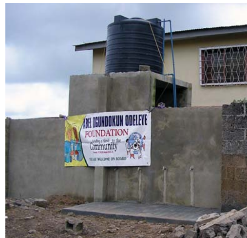
The water reservoir is fitted with four taps to reduce wait time.
