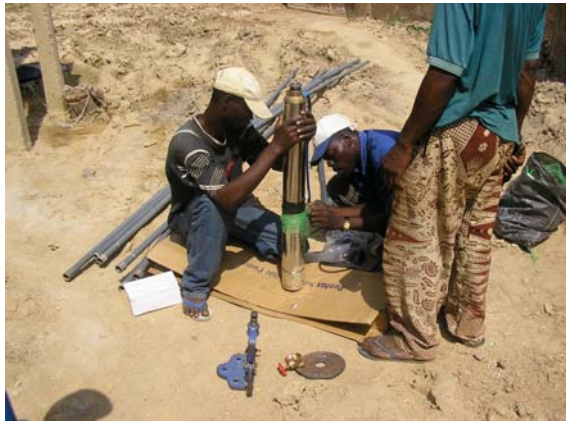
Workers hurdle as they work to sink the borehole pump.
